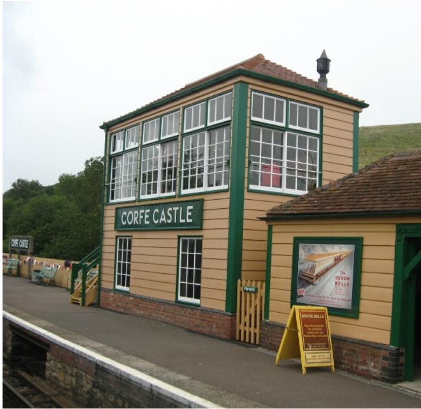
Above: Corfe Castle signal box.
